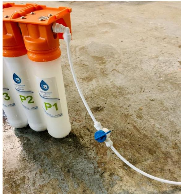
3. Connect the “new white ¼ nylon pipe that you received in the package to the pre filter side labeled “OUT”. Make sure you push the pipe all the way in. Some of the pre-filters do not come with elbows, those are not necessary.
